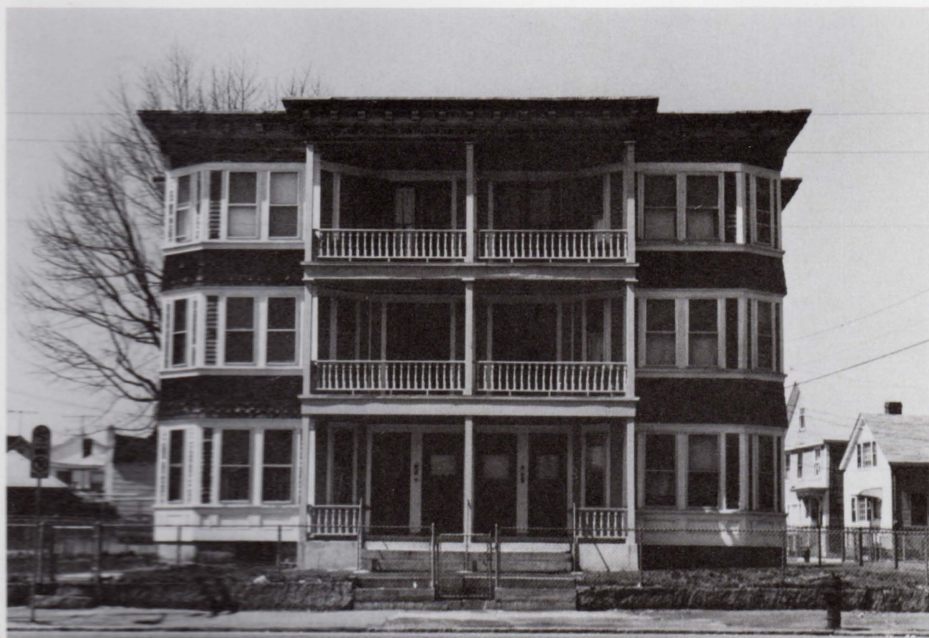
26. 621-27 Central St., ca. 1895. Three-decker buildings are rare on Chapel Hill because most of the available land was built up by the time they became popular elsewhere in Massachusetts. A few, with spacious floor plans and plentiful light, were constructed on Chapel Hill between 1880 and 1910. Double three-deckers, such as the one pictured above, contained six apartments, each with its own porch and bay window. The building has retained its original clapboard and shingle siding, dentil frieze and porch balustrades. It was built on the site of the Methodist Church, one of two early churches which lent Chapel Hill its name.
